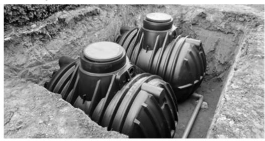
This is ideal for those who have limited space and want to keep their barrel out of sight. This type of water tank hence is expected to sit underground should be placed in a light traffic areas where heavy loads and vehicles are not regularly driven.
