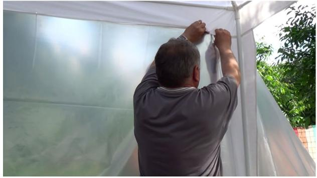
After you've finished connecting the foil to the roof, it's time to tie the corners. Run a plastic tie through the foil and around each pillar. 4 ties on each one will do just fine. Do it as you see in the video.
